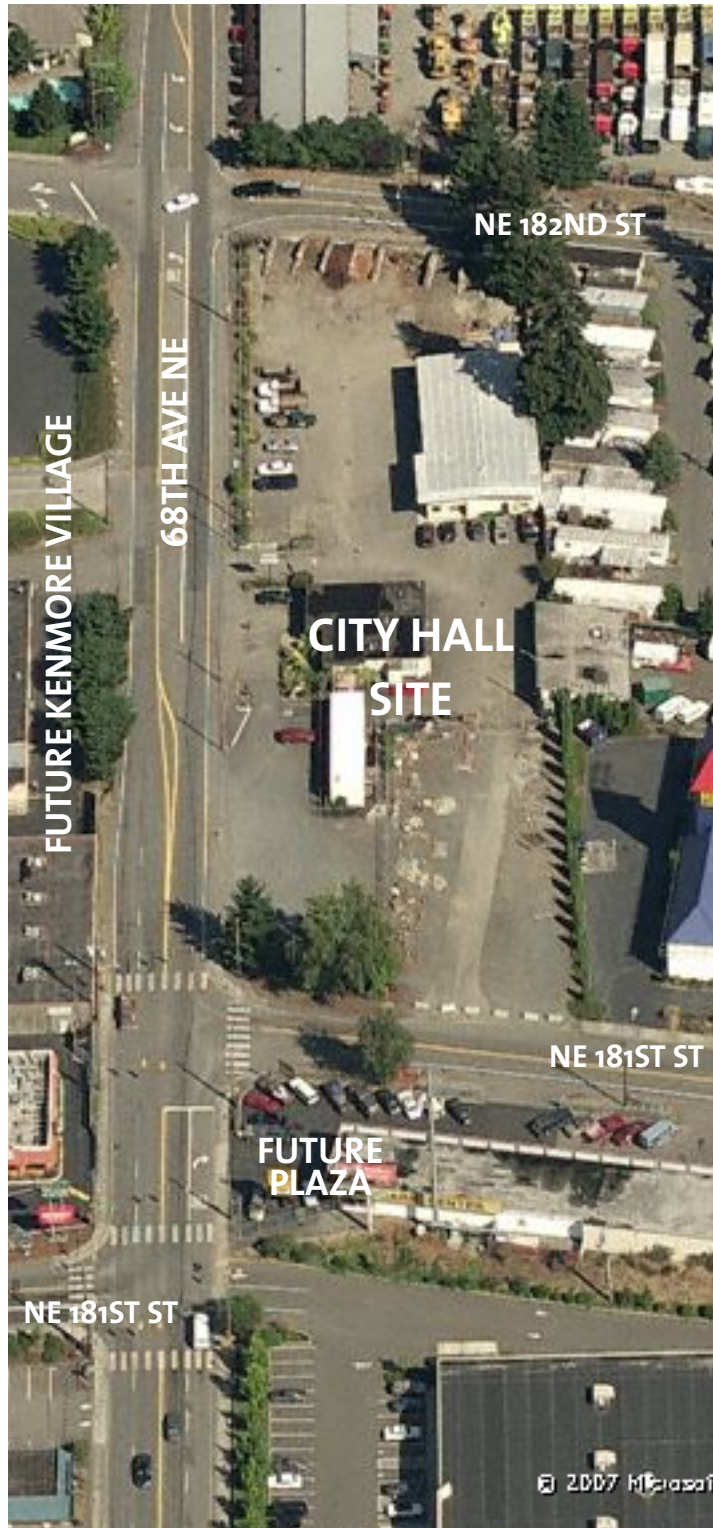
Aerial of City Hall site
